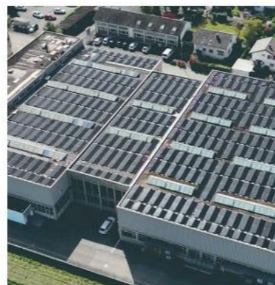
Switzerland Industrial and Commercial Rooftop Project
