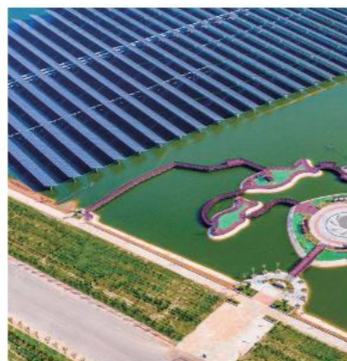
Shandong Dongying Yellow River Estuary Power Station
