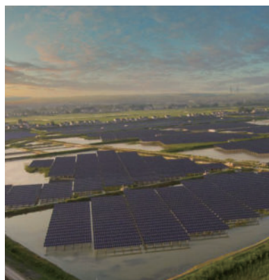
Jiangsu Nanjing Longpao Power Station
