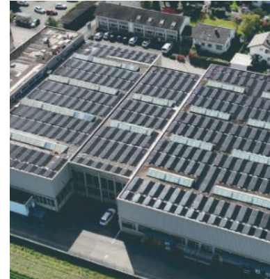
Switzerland Industrial and Commercial Rooftop Project
